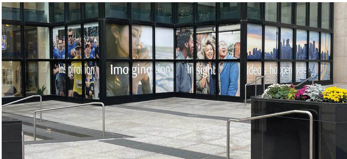
Royal Bank Plaza – South Tower, Toronto, Canada
