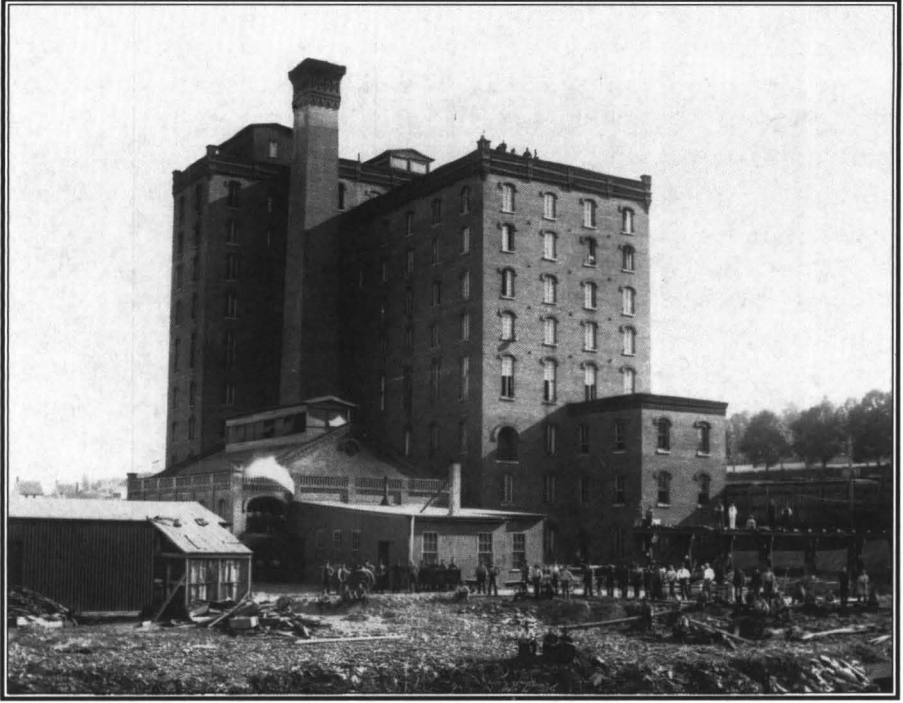
The Nova Scotia Sugar Refinery under construction in the early 1880s; “infant” industry arrives in Halifax.
