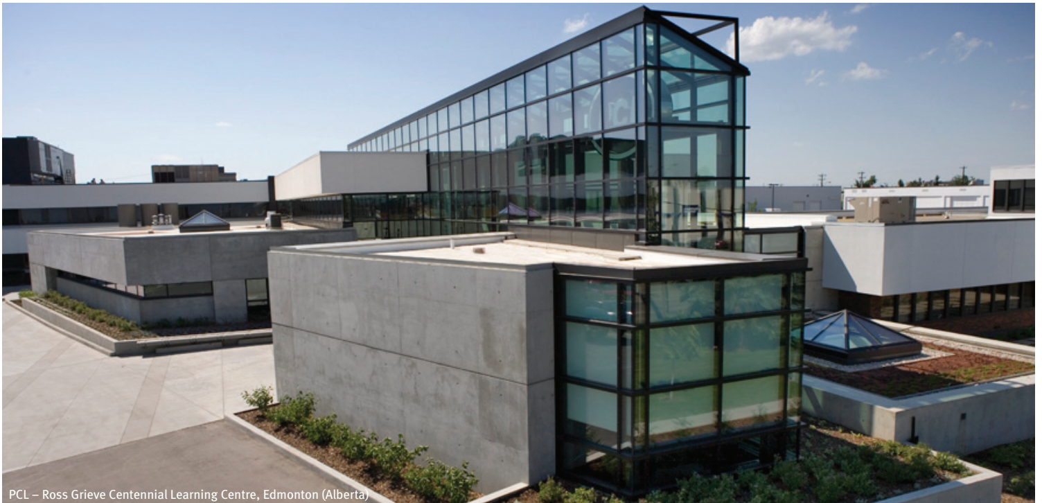
PCL – Ross Grieve Centennial Learning Centre, Edmonton (Alberta)
